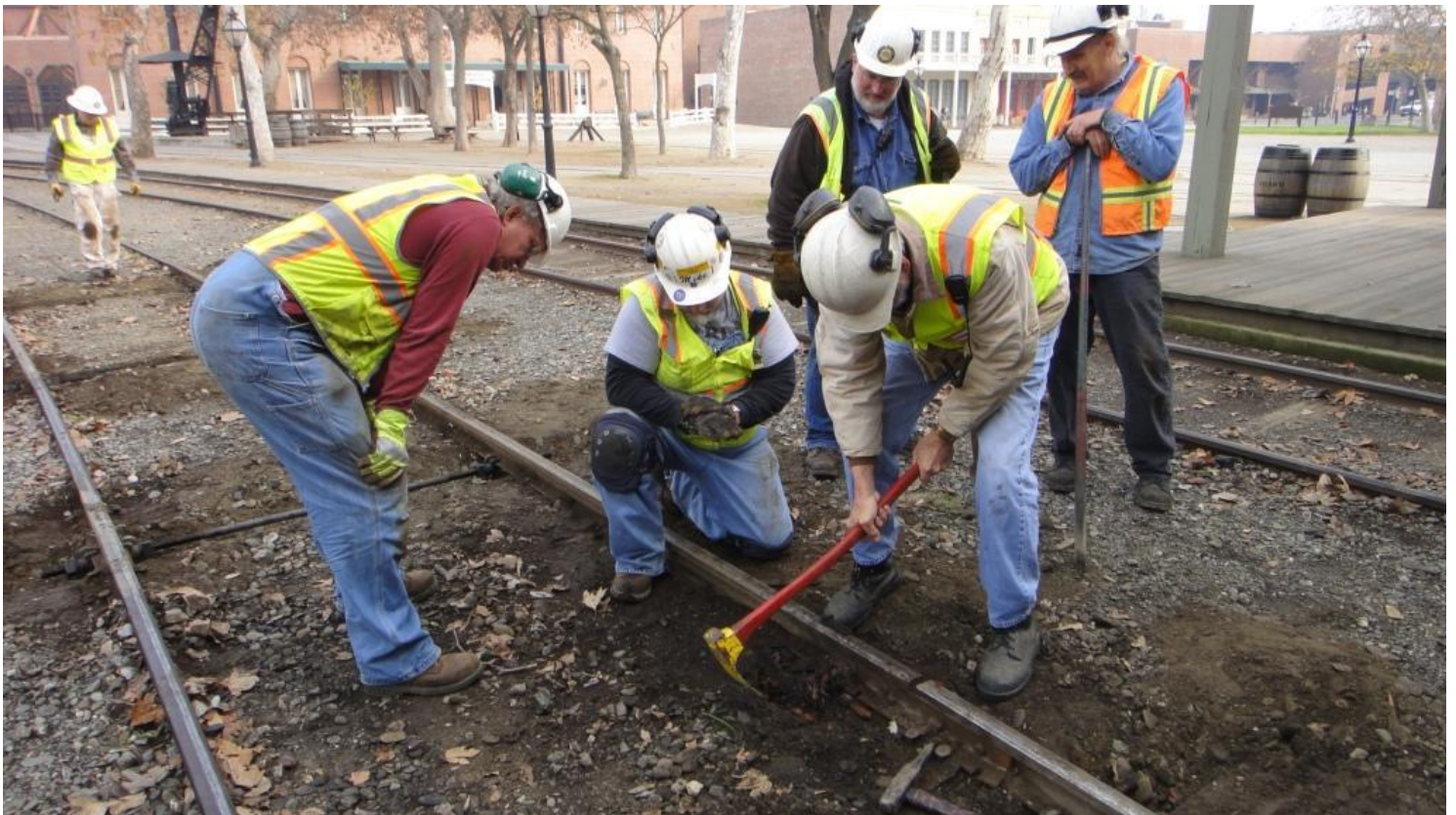
Because these redwood ties were pretty plate-cut, Alan brought in the adze to shave off the top of the tie so that the rail could be moved
