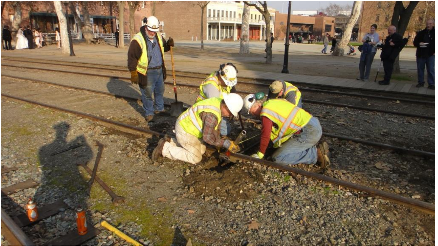
The MOW Team puts on a show as the fifth and final gauge-rod is installed
