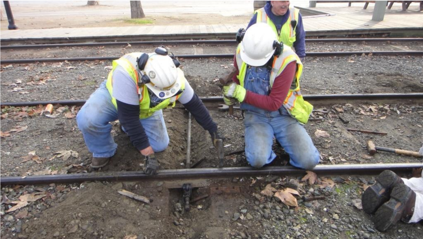
Mike F. and Steve plug the old spike-holes before the rail gauge is adjusted
