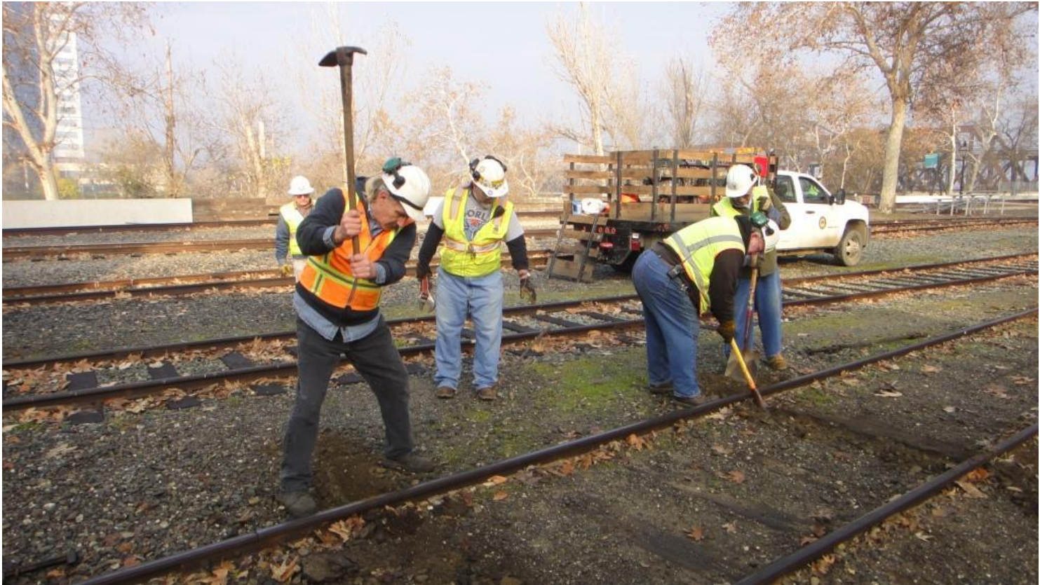
The Team gets to work on digging between the ties to insert gauge-rods on Track 2 into the CPPS
