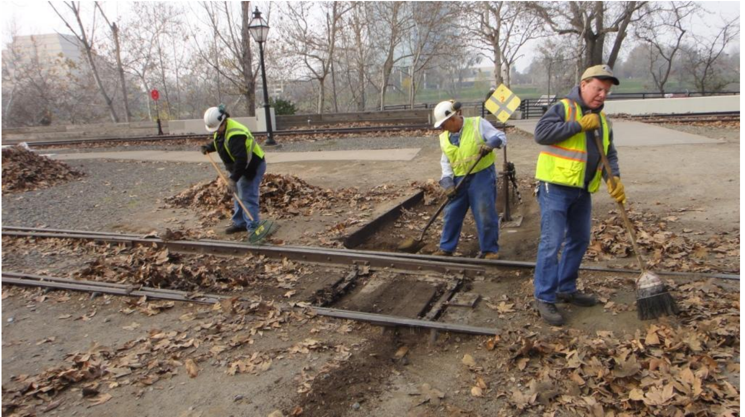
Heather, Clem, and Ed cleaned out Switch 2 which was buried in organic debris
