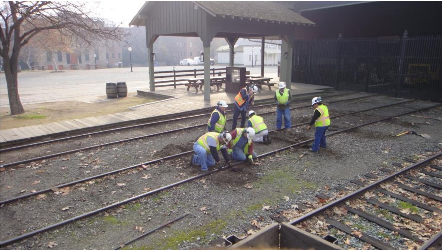
Your MOW Team at work installing five gauge-rods
