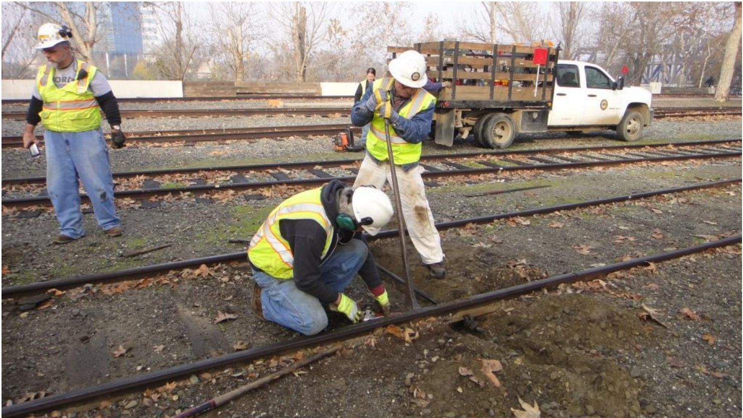
Steve and Mike H. pull spikes on the adjacent ties to allow for the lateral movement of the rail
